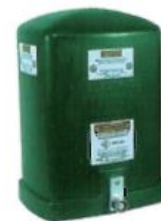
Typical secondary service pedestal
